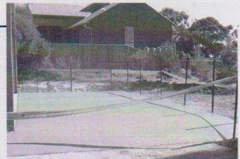
One of the new concrete slabs in 2010
